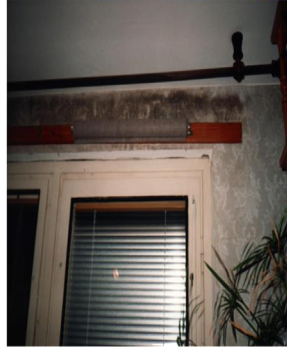
FIGURE 8 Continual vent opening causing cooling of the wall above, resulting in mold on it.
