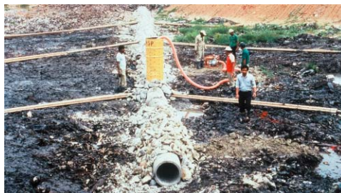
Photo 2-5 Structure of the Fukuoka method and its application in developing countries
