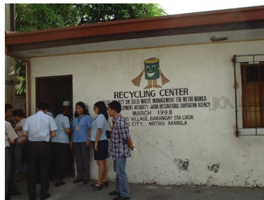
Photo 3-1 Recycling center constructed in the Soldier's Village in the P/P
