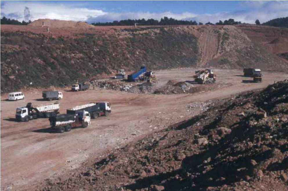
Fig. 1.12a Dumping construction materials (Metropolitan Environmental Organization, Barcelona).
