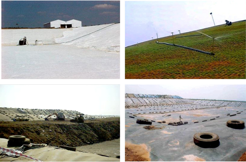
Figure 5.20 Treatment storage and disposal facility (TSDF). Courtesy: Ramky Group.
