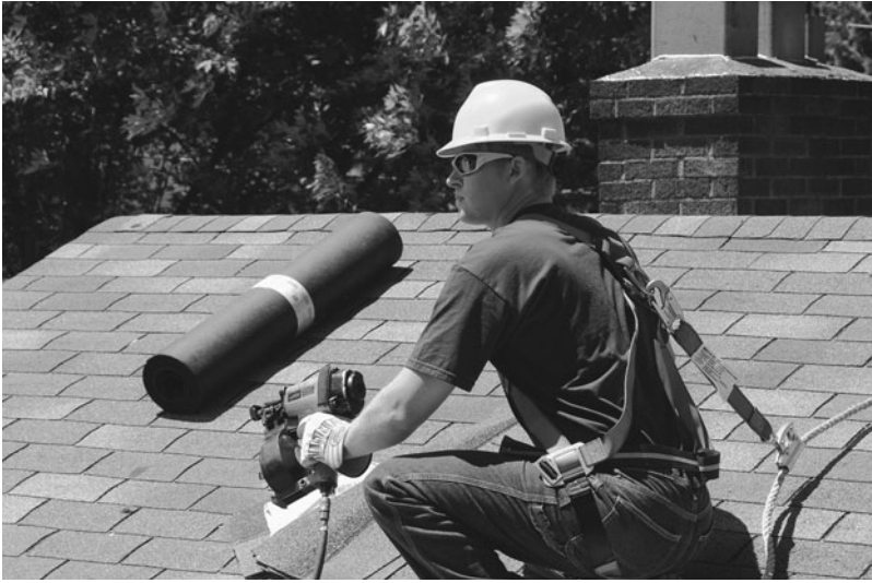
Figure 15-7. Worker wearing a full-body harness with attached lanyard properly tied off to a life line. (Photo courtesy of the Mine Safety Appliance Company.)
