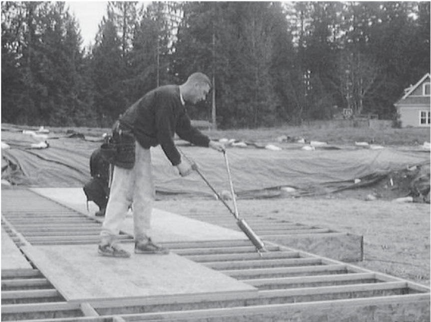
Figure 16-6. (A) Traditional method of applying glue to floor posts. (B) New method using commercially available extended gun ($50 retail). A handle was added to the gun to reduce hand/wrist fatigue (parts less than $10). Job times were the same for each of the two method. (Photographs by Barbara Silverstein.)
