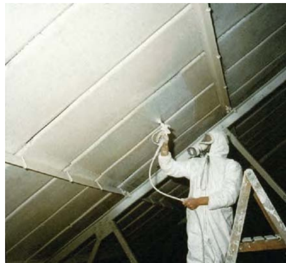
Figure 5.4 A lone worker – special arrangements are required.
