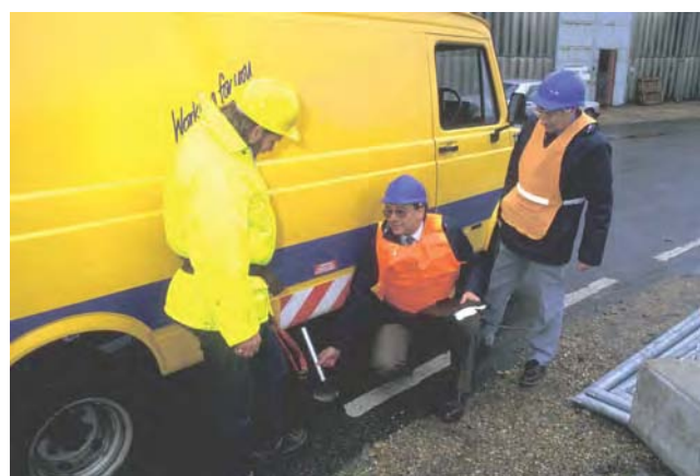
Figure 3.6 Contractors at work.
