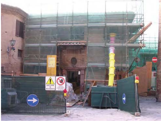
Figure 18.9 Construction site – Sienna.
