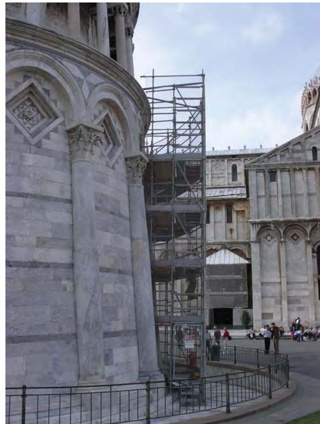
Figure 18.1 Good scaffold – Leaning tower, Pisa, Italy.
