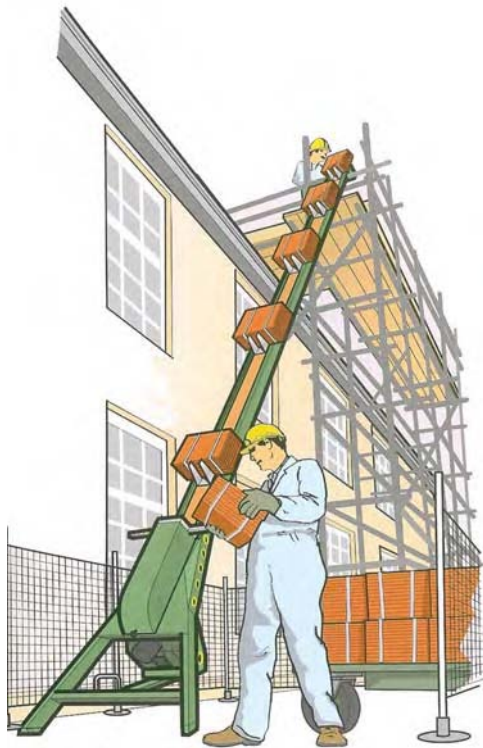
Figure 8.9 A brick elevator.
