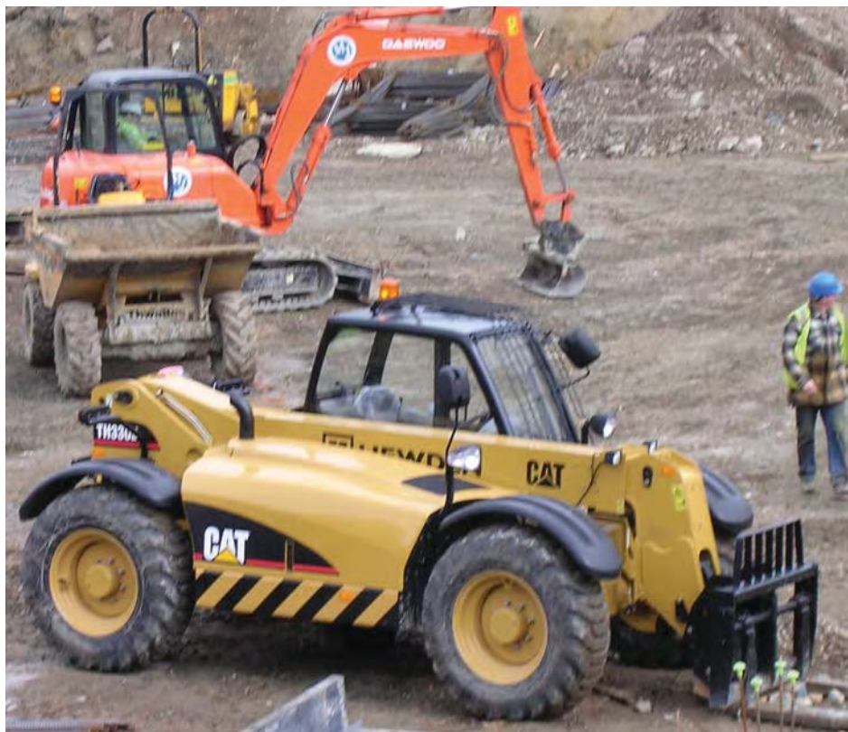
Figure 9.10 Various construction plant with driver protection.
