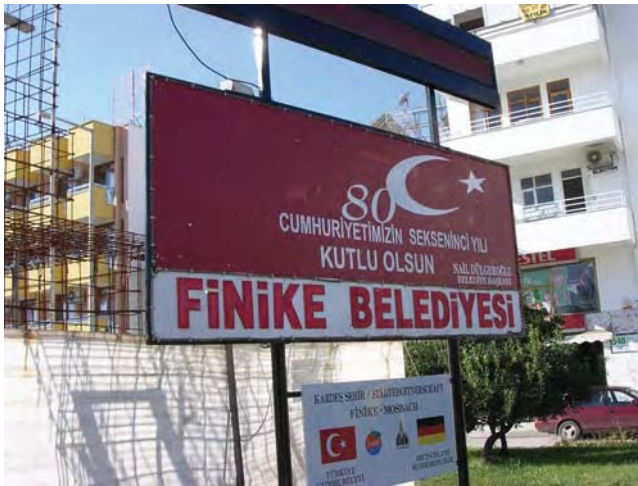
Figure 18.2 Local authority building site, Turkey.
