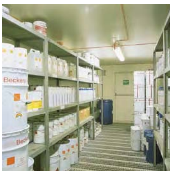
Figure 11.8 Various storage arrangements for highly flammable liquids.
