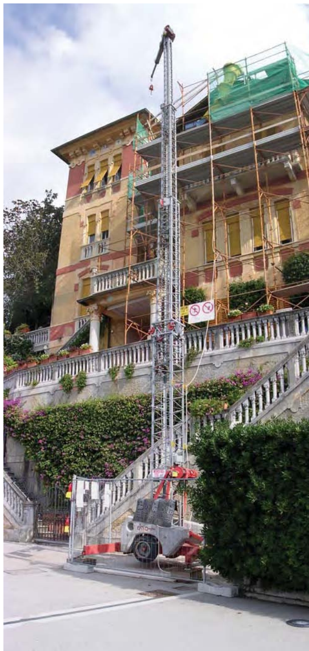
Figure 18.12 Mobile tower crane – Cinque Terre, Italy.
