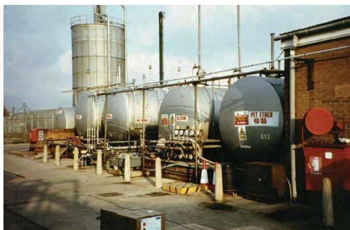
Figure 7.4 (a) Typical warehouse vehicle loading/unloading area with separate pedestrian access; (b) barriers to prevent collision with tank surrounds/bunds.
