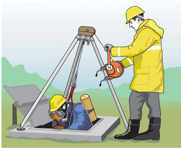
Figure 6.9 Entering a confined space.
