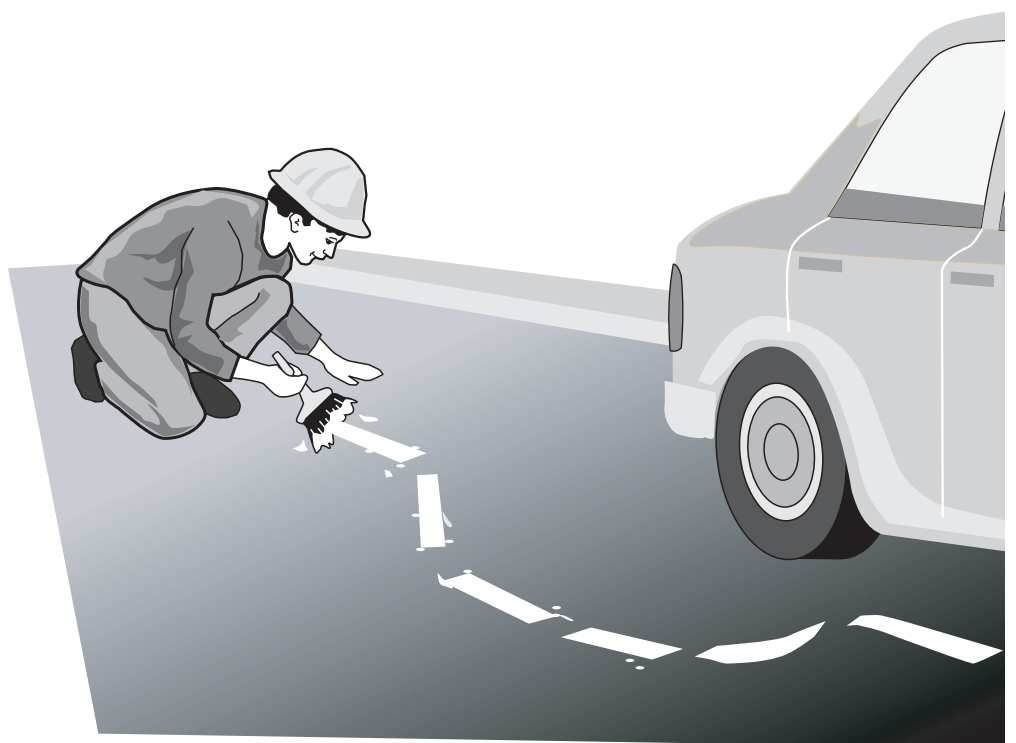
Figure 13.13 Help needed here.
