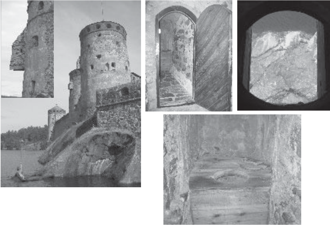
Figure 4.12 Bay privies attached to towers (Olavinlinna castle, Finland), entrance, the scenery downwards and the seat (constructed later). (Photo: Petri Juuti)
