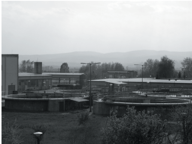
Figure 25.3 The wastewater plant of Miskolc with mechanical treatment was constructed in 1972. (Photo:Viktor Pál)
