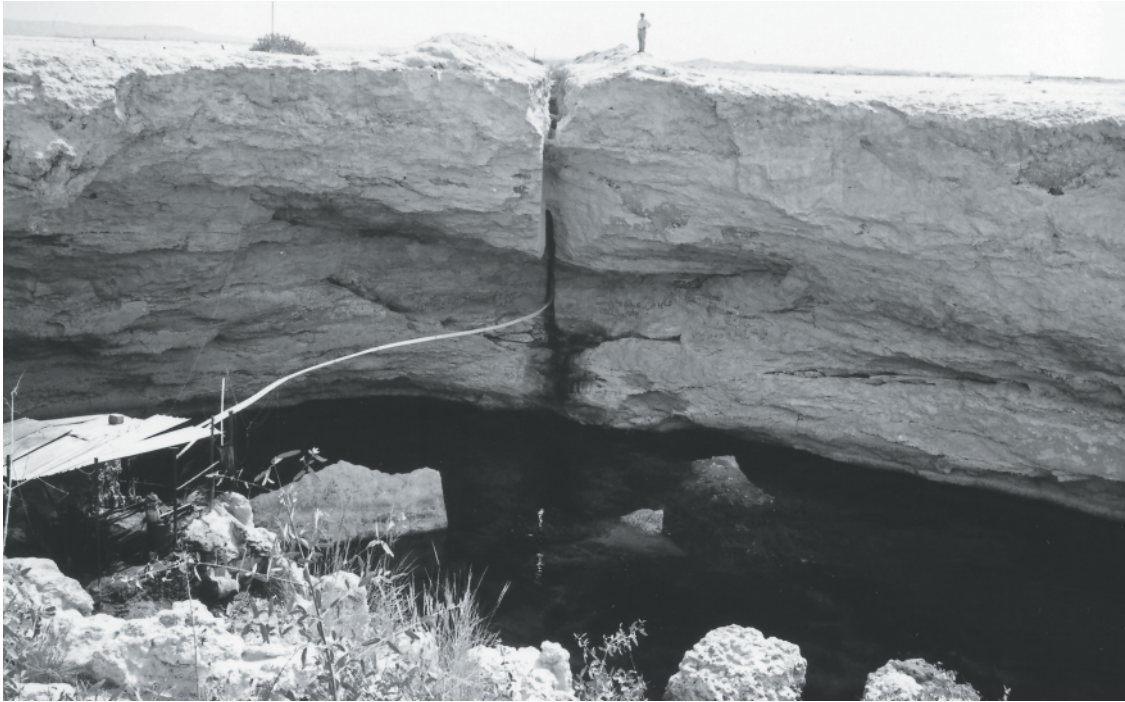
Figure 15.8 Water pumped from a collapse sink is fed into the existing underground channel network.
