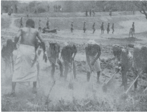
Figure 22.8 A gang of villagers digging a spill-way.
