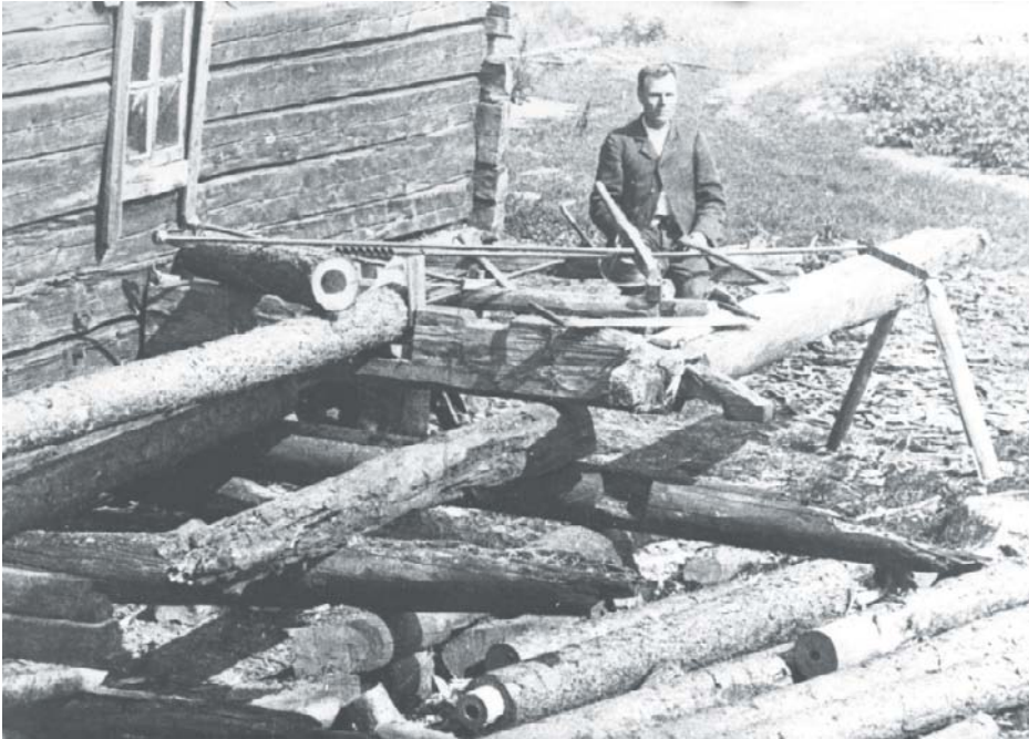
Figure 24.2 A manual driller of water pipes made of pine wood in 1913 in Sumiainen, Central Finland. (Photo: Vanhan Äänekosken kotiseutuyhdistys.)
