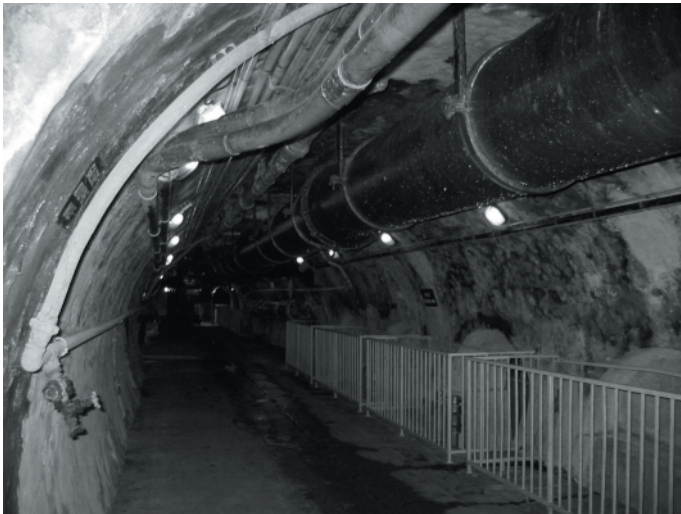
Figure 33.2 View from Paris sewers. Note oval shape in smaller sewer. (Photo: Petri Juuti)
