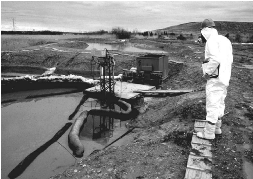
FIGURE 19.8. LEACHATE COLLECTION PONDS AT THE KIN-BUC LANDFILL IN EDISON, NEW JERSEY.
