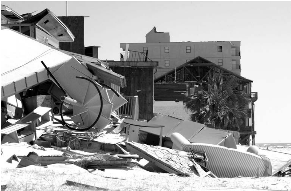
FIGURE 26.2. DEBRIS AND DAMAGED BUILDINGS IN PENSACOLA, FLORIDA, RESULTING FROM HURRICANE IVAN, SEPTEMBER 2004.
